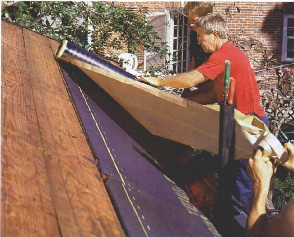
Thwarting ice dams. To get a watertight seal that protects against leaks caused by ice dams, use Ice & Water Shield. It sticks to the sheathing because it's coated on one side with adhesive. Put a single layer of it at the edge of the roof over the bottom drip edge before papering in. Some roofers will even run Ice & Water Shield in valleys for added leak prevention.
